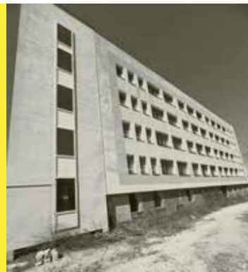
Unfinished building of PHI General Hospital Kičevo
