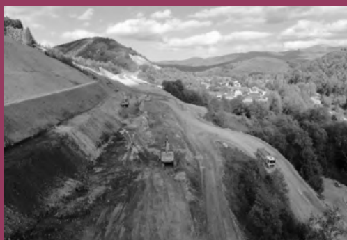
Rehabilitation activities on a landslide on Kicevo - Ohrid road section
