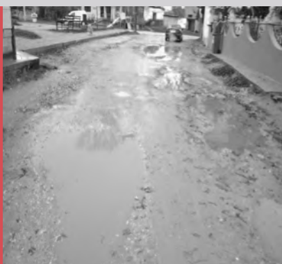
Infrastructure in rural area, village Furka, near Dojran
